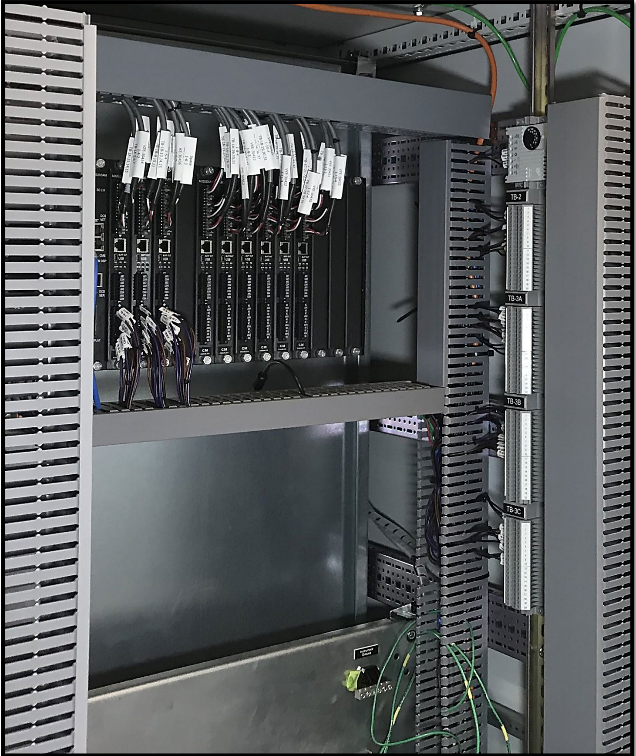
Figure 1: Best Practice VC-8000 Installation 16 position rack, bulkhead mounted to subpanel
